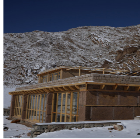
Pre-FREB (Fibre-Reinforced Earthen Blocks) building, a technique in which the entire construction is pre-fabricated and assembled on site, making construction twice as faster.
