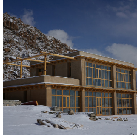
It is a wall building technique used by ramming the earth in a pre-fabricated mould.
