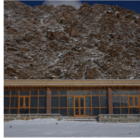
Bricks made of straw & clay are used, replacing the traditional bricks.
